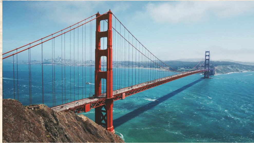
Golden Gate Bridge San Francisco
